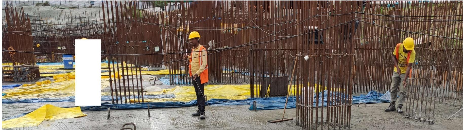
Column rebars forming Shear-keys in Raft
